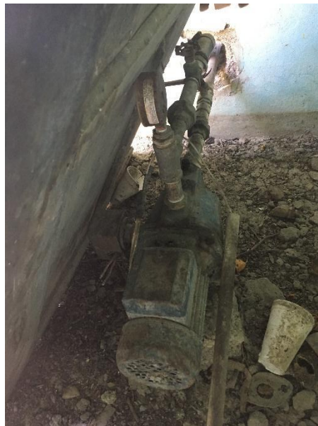
Figure 1-14 – Abandoned Tank Circulator Pump
