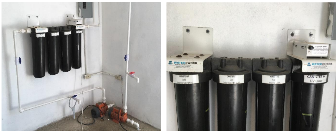
Figure 1-17 – Bottling Plant Treatment Equipment
