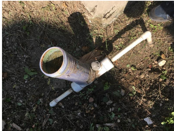
Figure 1-16 – Chlorinator Unit
